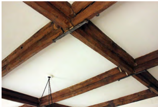
Moulded ceiling beams
