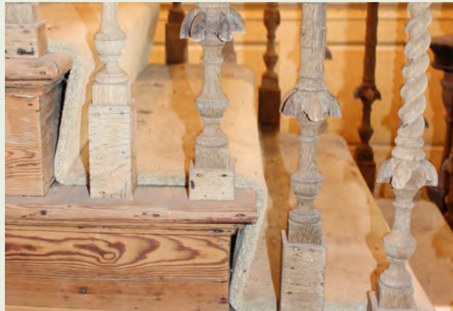
Detail of base of balusters and plain tread ends
