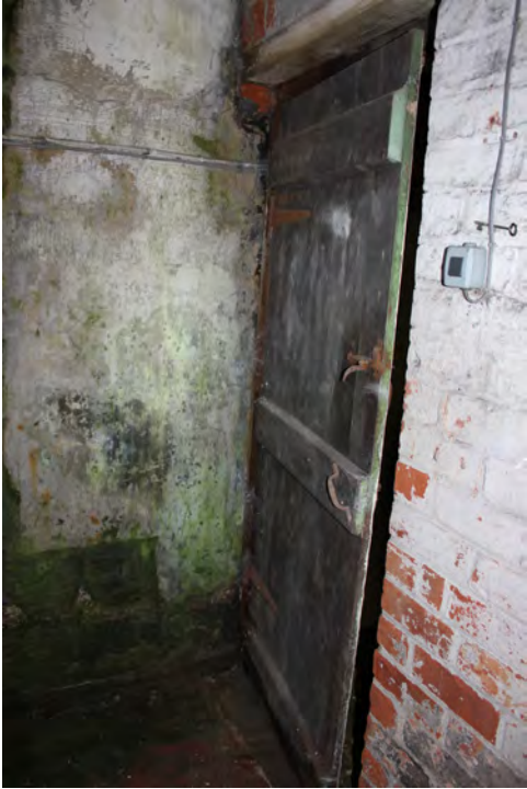
Timber ledged and braced door
