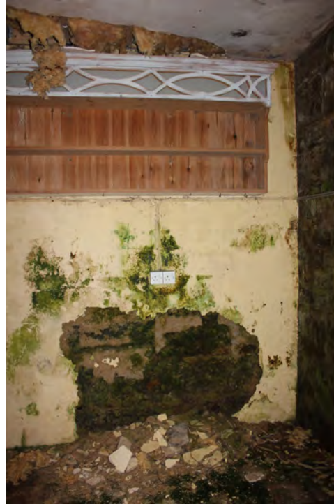
East wall - eroded plaster reveals stone wall behind
