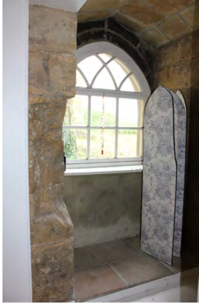
Window inserted into medieval doorway
