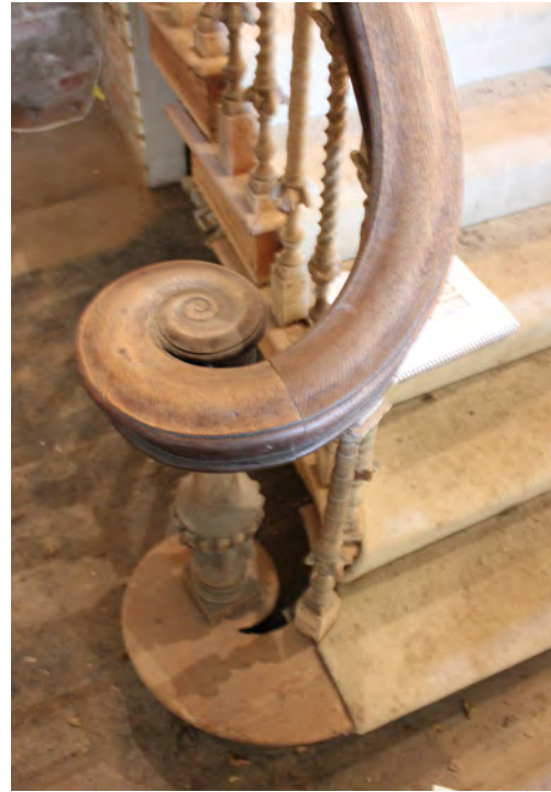
An absence of balusters at the curtail
