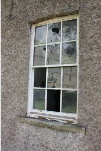
Timber sash window in western elevation
