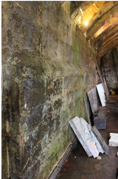
Chamfered plinth to north wall
