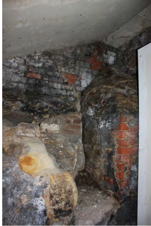
North wall – a combination of stone and brick
