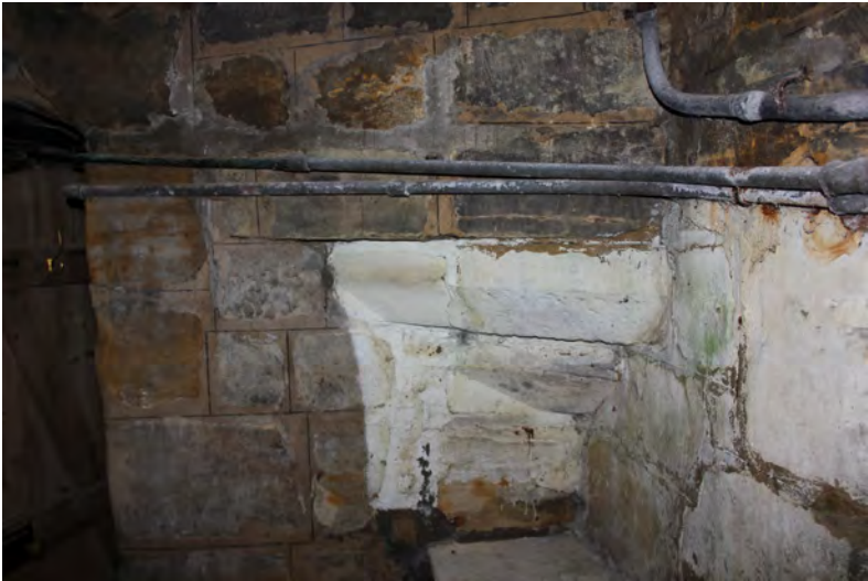
Painted corbelled base possibly of the former spiral stair in adjacent space
