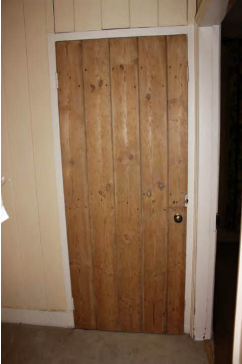
Ledged and braced door
