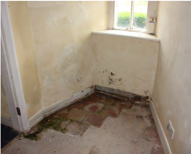
Quarry tile and concrete floor
