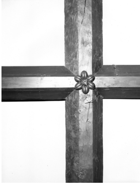
Detail of ceiling – note the modern beam intersects from the left and right
