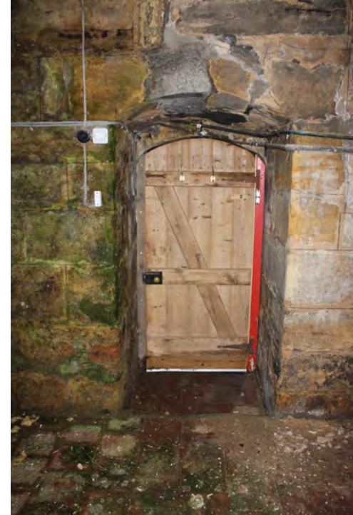
Timber ledged and braced door to Kitchen
