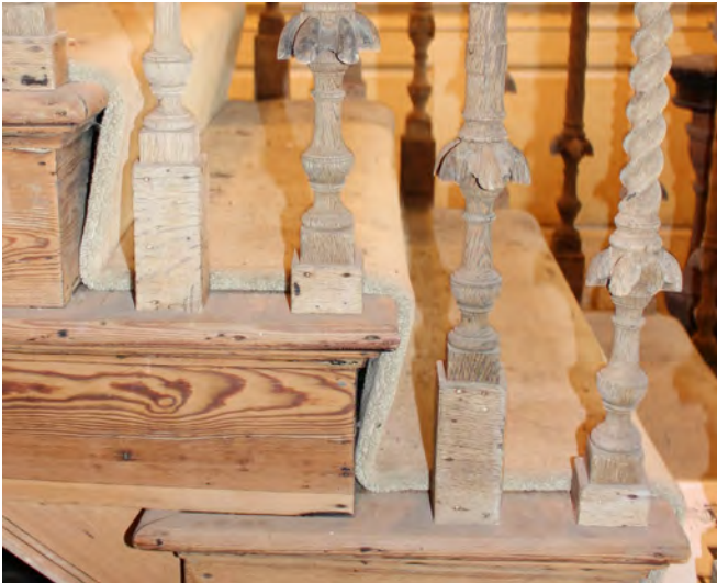
Detail of base of balusters and plain tread ends
